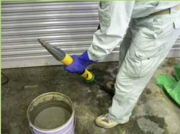
**Quickly Rotate pump above 45° to stop grout flowing out**
