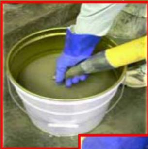
**Empty and Flush grout from pump thoroughly
