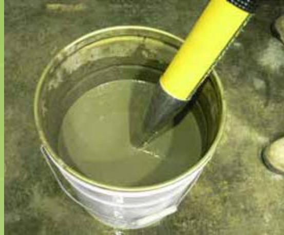
Inserting the nozzle cap well beneath the surface of the Nissco SS Mortar,
