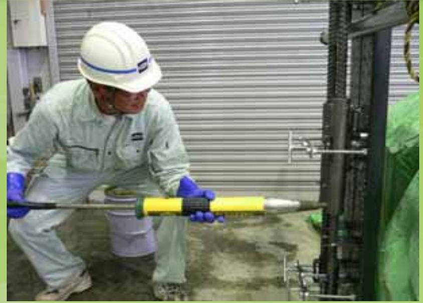
For Vertical Sleeves Keeping the Handy pump on as much of an angle as possible, Insert (45° cut) Nozzle Tip into the grout tube then quickly rotate it to the horizontal position pushing the plastic Nozzle Tip firmly into the PVC tube to make a good seal.
