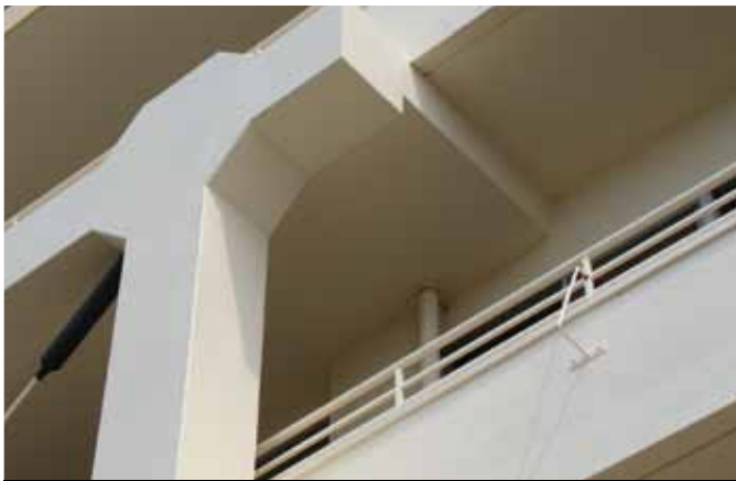
Figure 3. Cast-in-place concrete diaphragm of retrofit of Shiogama Municipal No. 2 Junior High School.
