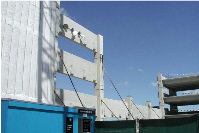
Logan Airport Garage Under Construction
