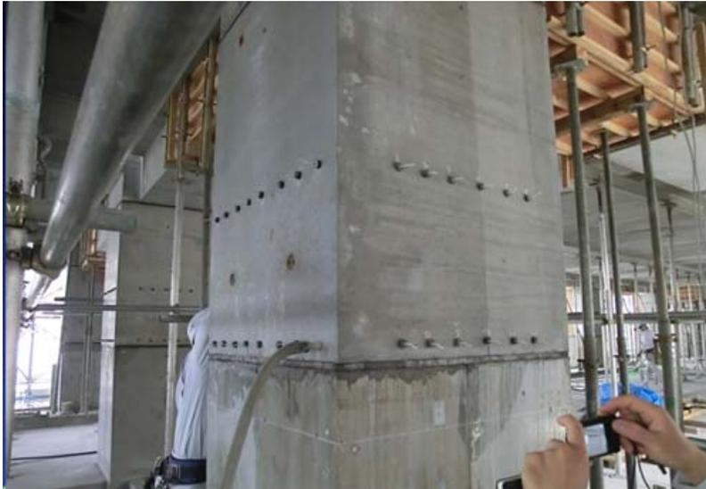
NMB Splice Sleeve's grouting crews have developed and perfected the specialized Mass Grouting procedures, equipment and gadgets overseas. They have successfully performed Mass Grouting for many years to the point where it is now an industry standard procedure in Japan. Splice Sleeve North America intends to offer training in these procedures for professional grout crews during 2013. For more information, please [contact Splice Sleeve North America, Inc.](#)
